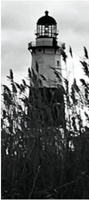
Montauk Point Lighthouse
